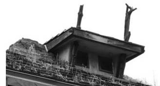
Fig.10 Tanpopo House, piercing columns executed only at the 2nd story window canopy
