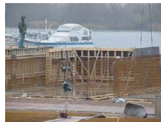
Fig. 23 Construction on Site for Gouden Kust Housing
