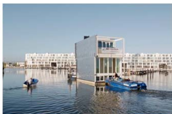
Fig. 5 Towing the Modular House
