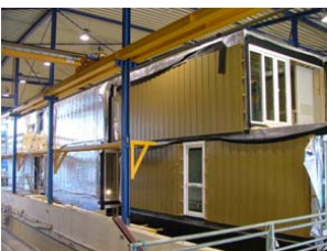
Fig. 4 Under Construction in the Dry Dock
