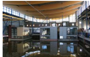
Fig. 21 Under Construction for Terwijde Housing
