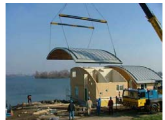
Fig. 24 Construction on Site for Gouden Kust Housing
