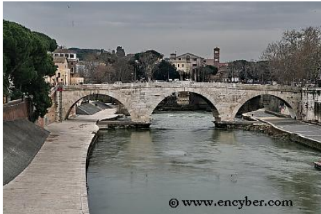
Fig. 3 The Pons Cestius bridge (BC62~BC27) in Rome, Italy[Photo:http://100.naver.com/100.nhn?docid=925898]
