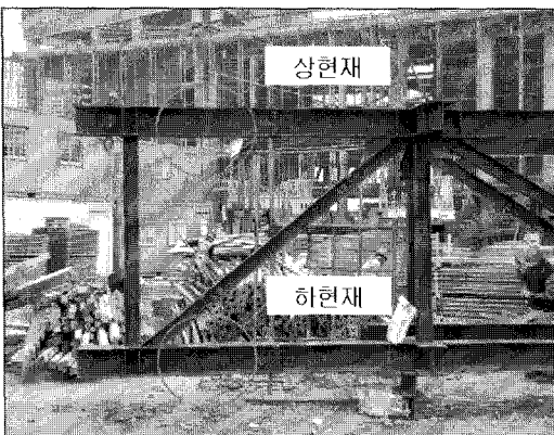
Fig. 8 Roof truss upper and lower chords
