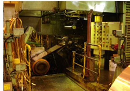
Fig. 14 6 high-mill for thin cold rolling process
