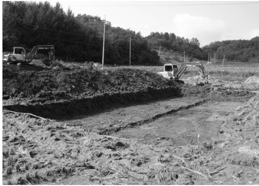
1) Surface soil removal
