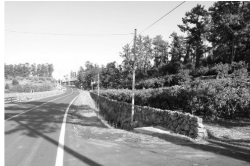
After the extension of a road(2010)
