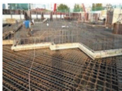
(e) Transfer Mat 형틀/철근
