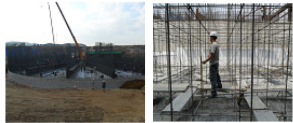
(a) Construction site
