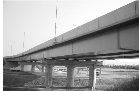
Fig. 15 The Target Bridge for Communication Test
