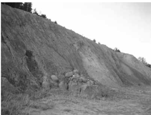
Fig. 1. Typical slope developed in granite (Site A).
