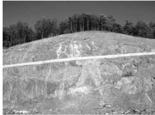
Fig. 2. Typical slope developed in granitic gneiss (Site B).
