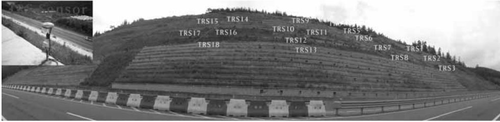
Fig. 15. Installation of Translation-Rotation-Settlement sensors.
