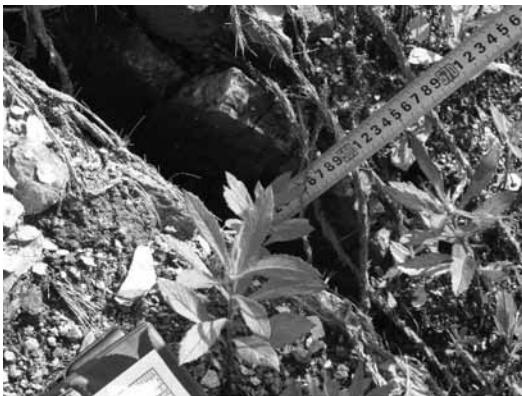
Fig. 6. Observation of tension cracks (July 2007).
