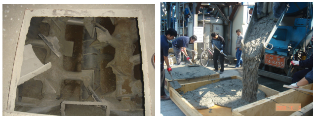
(a) 2-Shaft mixer_3500 L (batch) (b) Placing in Mock-up
