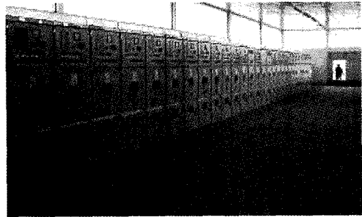
Switching Station 중심개폐소
