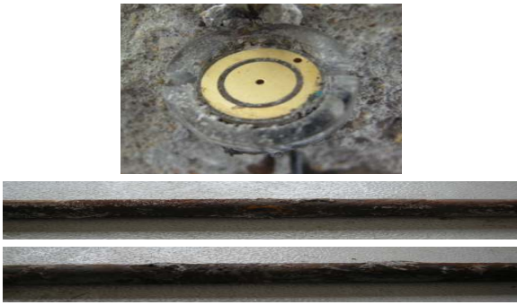
Fig. 7 The status of rebar and mini-sensor after end of experiment
