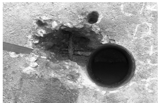
Fig. 1 Measurement of carbonation depth
