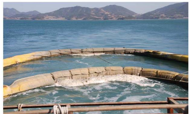
Fig. 10. Gathered foam at the outlet of the discharge channel before(left) and after(right) the installation of TTPs.
