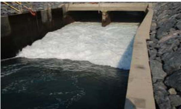
Fig. 4. Generation of foam at the discharge channel.
