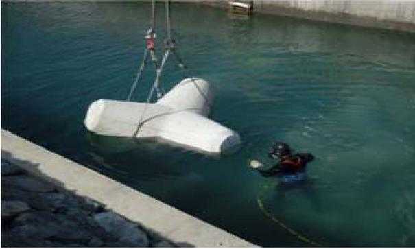
Fig. 8. Installation of TTP at the discharge channel.
