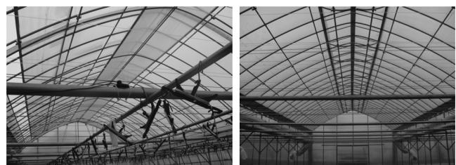
(a) Rollup type vent at eave (b) Butterfly type vent at ridge
