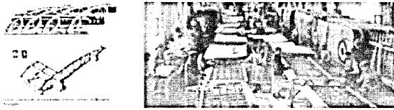
a) Wing construction b) Ansaldo Aircraft Factory(1920's)
