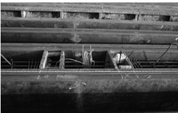
Fig. 3 Thermocouple wires for concrete piles.
