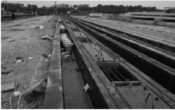
Fig. 2 Cylinders and finished piles with embedded shrinkage plates.
