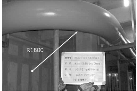
[그림 8] Photos of curved pipe for a refuse collection system
