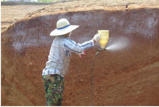
Figure 2. Spray using a mortar gun.
