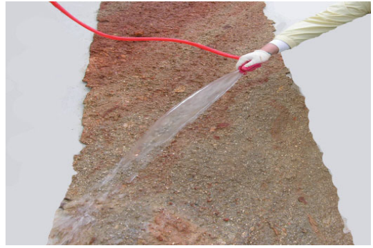
Figure 7. Wash the surface of soil layer.
