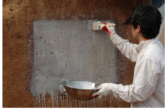
Figure 3. Coating using common brush.
