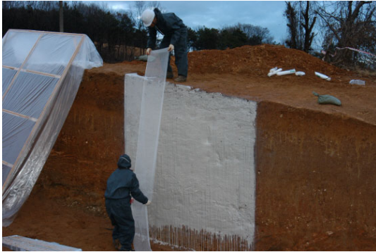
Figure 4. Attach primary gauze.
