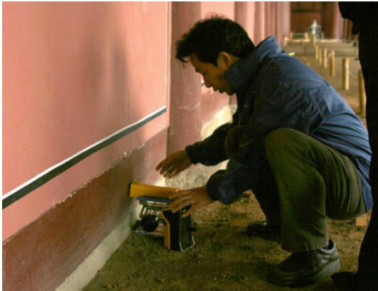
Figure 5. Detecting termites in wooden structure.
