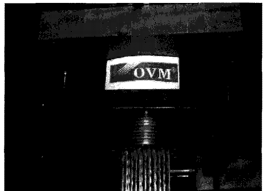
Fig. 7. Bottom anchorage anchor head.
