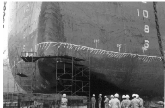
Fig. 7 Bow damage of single hull VLCC due to grounding
