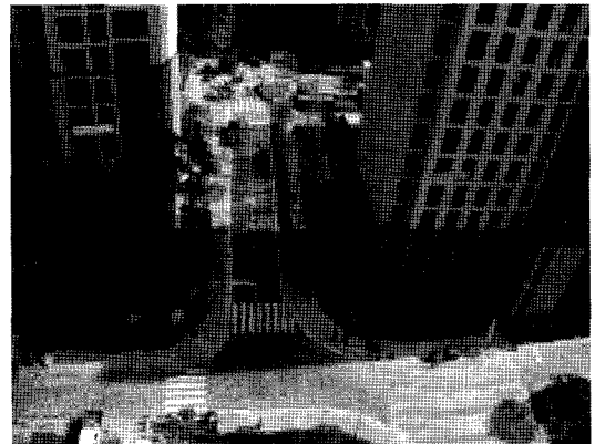
Fig. 2 The Road Snow-melting system is reclaimed at this actual area
