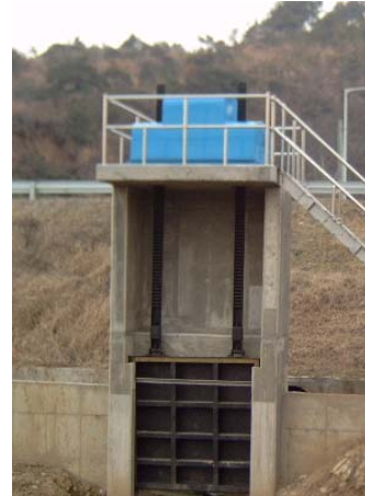
Fig. 1 Rack-bar type sluice gate applying the electric motor, worm gear and gear speed reducer
