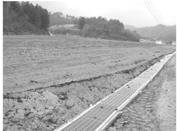
(b) Drainage Ditch
