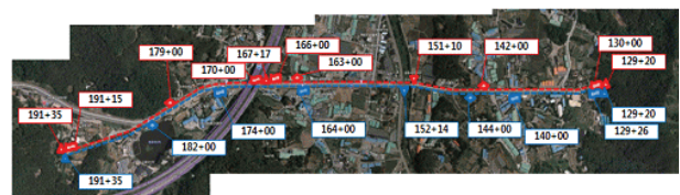
Fig. 2. 2 tunnel exit~3 tunnel entrance
