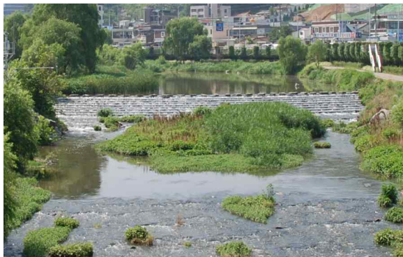
Fig. 1. Stepped Weir in Field
