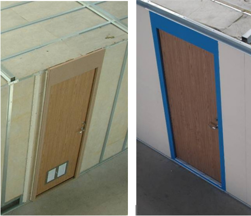
(a) Original door (b) High noise reduction door
