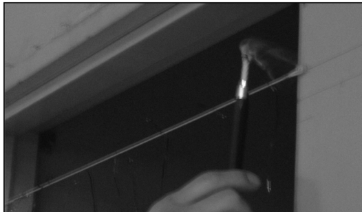
Figure 3. Backflow test by the smoke tester.
