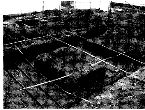
Fig. 2 The laying view of the pipe lines.
