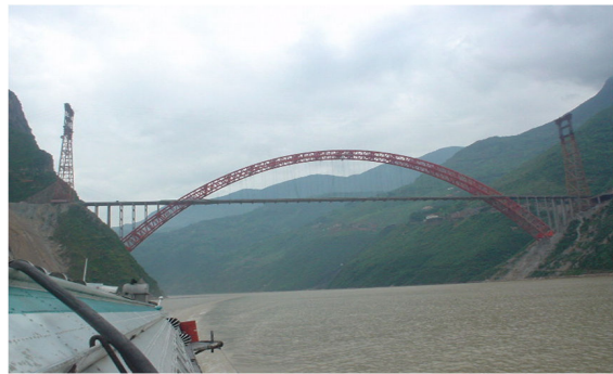
사진 4. Wushan Changjiang River Bridge
