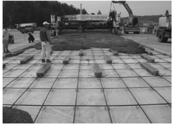
Fig 1. Concrete placement in field.
