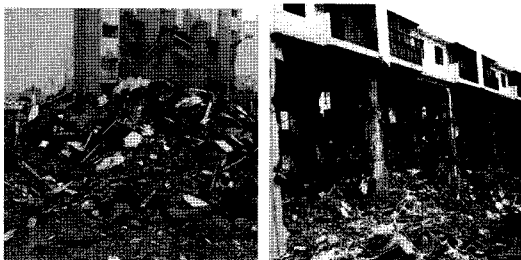
Photo 1. Increasing construction waste by dismantling structures.
