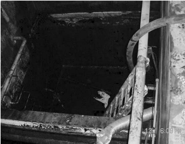
Fig. 1. Pond room(2.5 m×2.2 m×3.2 m). A hose of tank lorry and a ladder were set up.
