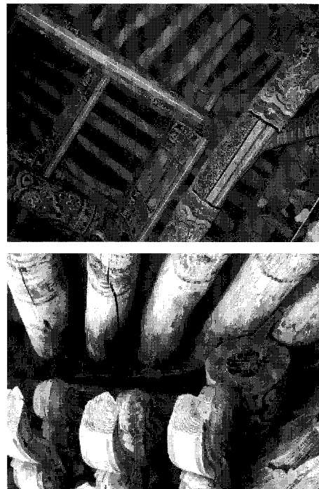
Fig. 7 the state of the roof
