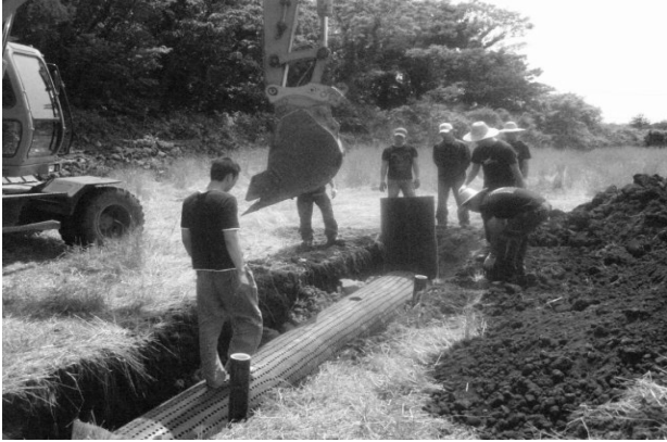
Fig. 11. Installation of infiltration trench in field
