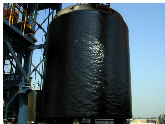
Fig. 4. Coated PCCP pipeline
