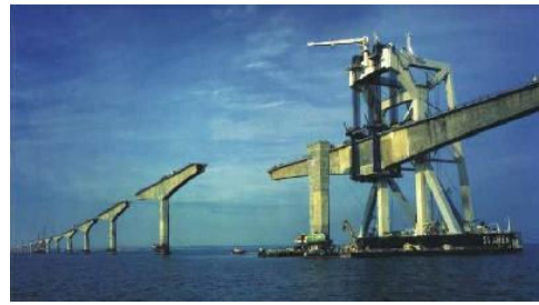
(a) Confederation Bridge(Canada)
