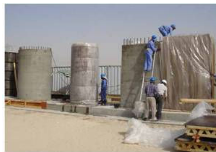
Fig. 6 Heat of hydration mockup test
