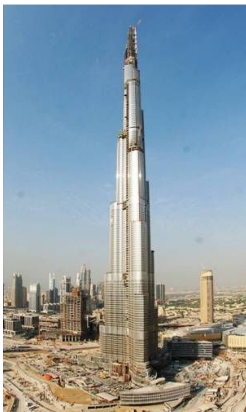
Fig. 8 Construction progress photos
