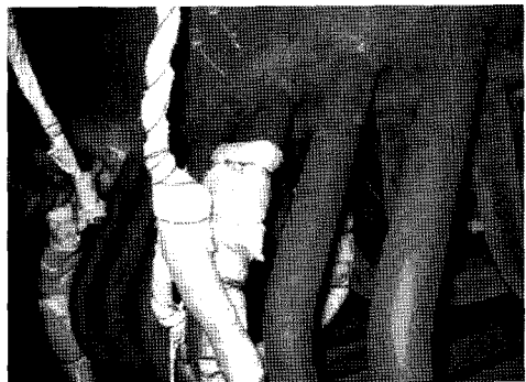
(b) Attached thermocouples on tubes
