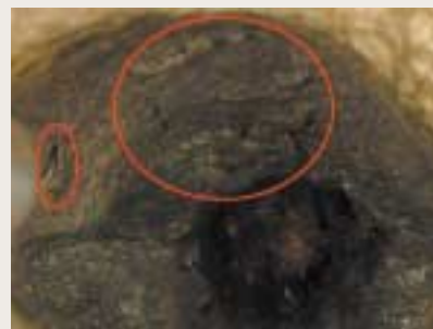
(b) Casting defects(scab)
