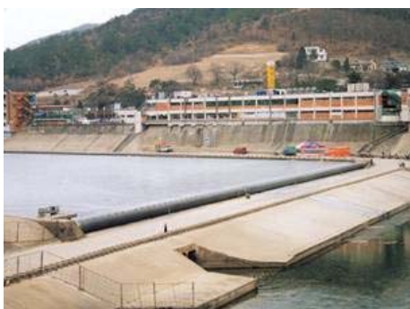
(a) Rubber dam for small hydropower
