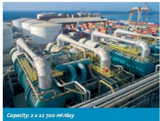
**Fig. 2 MED-TVC desalination plant. This photo is cited from the Sidem's catalogue[4].**
