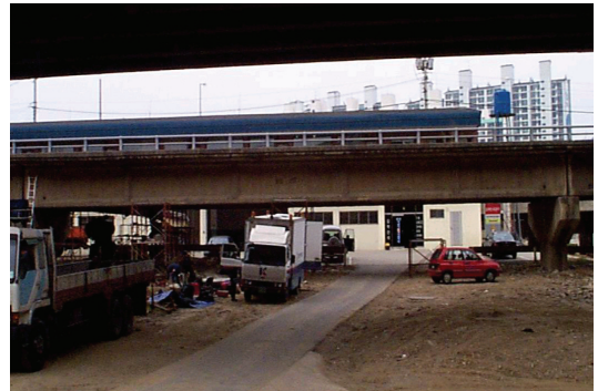
Photo 1 The PSC I-Typed girder bridge
