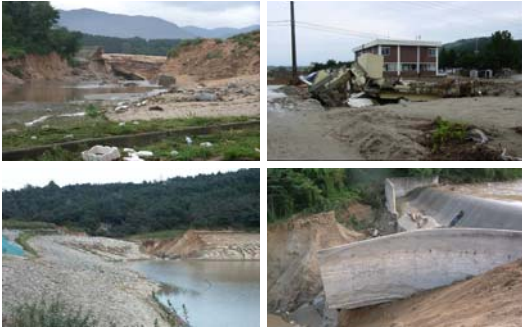
Fig. 2 Dam failure caused by Typhoon Rusa in 2002; (a) Dam body failure on the left abutment of the reservoir, (b) Damage to downstream area due to the collapse of the reservoir (c) Collapse of the dam body and spillway out of the Dam, (d) Collapse of the spillway foundation and the spillway
