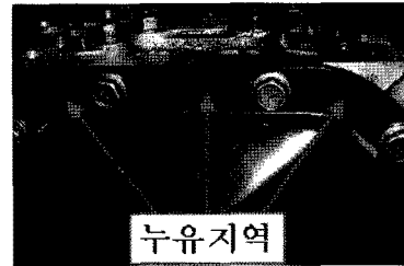
Fig. 4. Oil leakage and sealant sealing.
