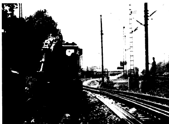
Fig. 2 Working Gang with Heavy Construction Machine on a Two-track Line while the Traffic Regularly Goes on [2]
