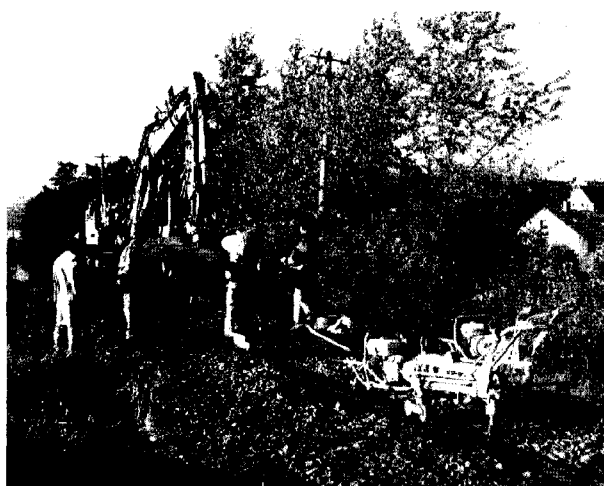
Fig. 1 Working Situation of Gang Workers on a Railway Construction Site [1]
