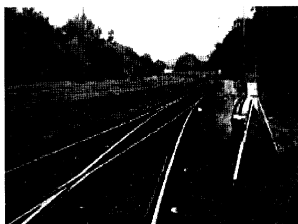
Fig. 3 Security Staff for the Warning of Gang Workers in Front or in the Rear of the Construction Site [3]
